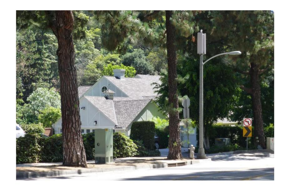
This small cell deployment features antennas that are under 3 cubic feet. Supporting equipment is housed at ground level in a 22½ cubic foot cabinet
